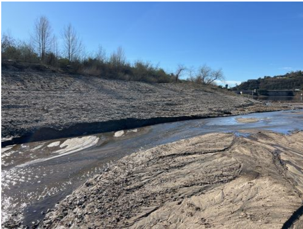
Erosion_along_toe_of_slope_E_side.jpg -118.17241043055556 34.192032491666666
